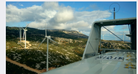
Goritsa, 33.3 MW power station commissioned in 2017 in Greece.
