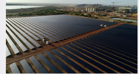
Essakane Solar, a 15 MWc solar power station commissioned in 2018 in Burkina Faso and serving the Essakane gold mine.
