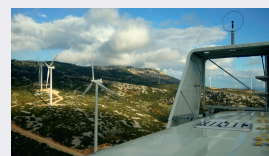
Goritsa, 33.3 MW power station commissioned in 2017 in Greece.
