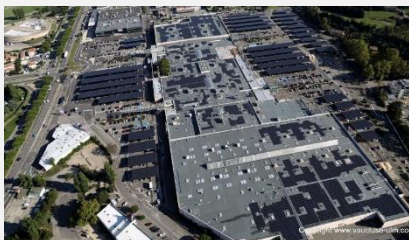
Energy Generation (build / sell model of decentralized photovoltaic plants on retail/ tertiary sites)
